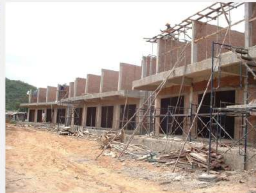
Structural Steel Framing
